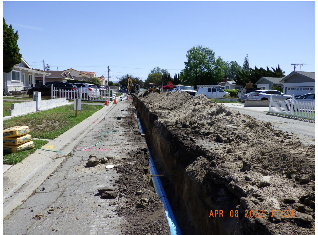
Water Main Replacement Alwood Ave-Anthony Ave (4,200 lf)
