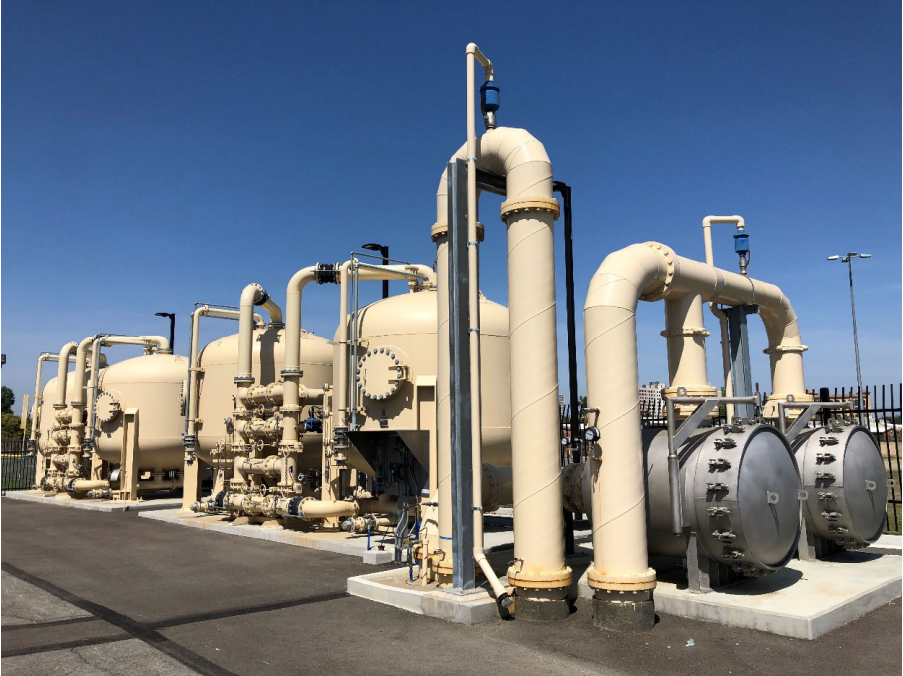
PFAS Equipment at the Westhaven Reservoir
