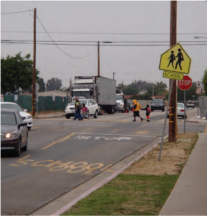
Faded pavement markings along Kerry Street and 11th Street.
