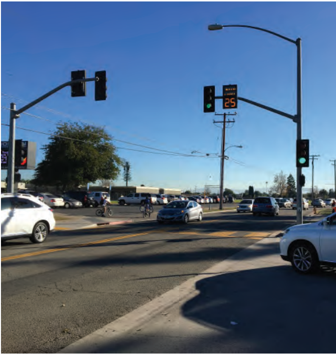
Traffic signal with mid-block crossing immediately in front of Cook Elementary.
