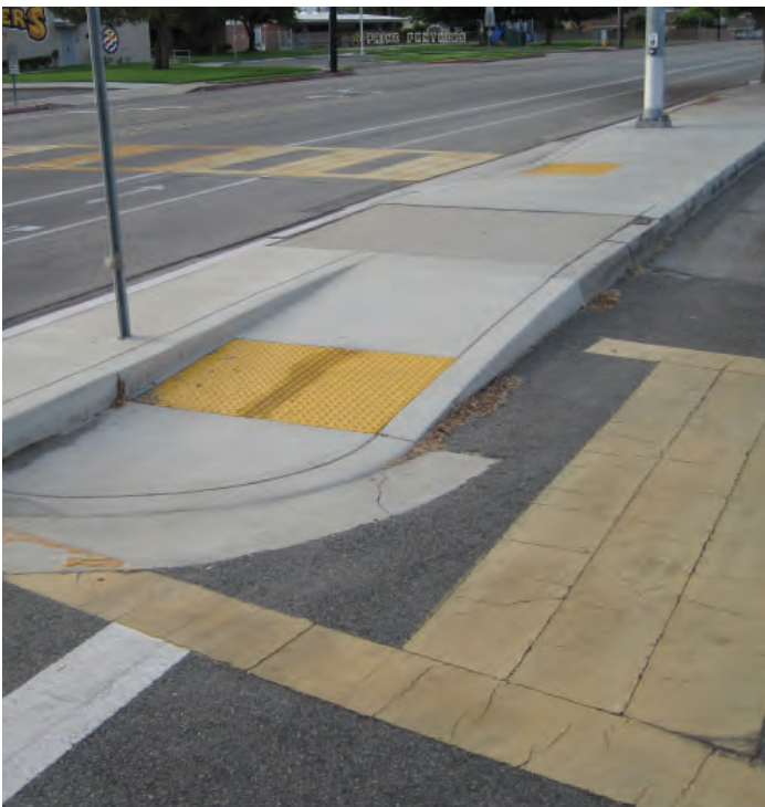
ADA compliant curb ramps provided at existing pedestrian signal crossing and adjacent roadway.
