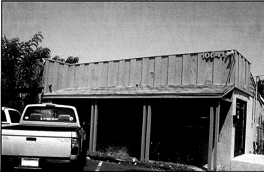
View of vacant business along the Garden Grove Blvd. frontage (10641 Garden Grove Blvd.). This building will be demolished to accommodate the project.
